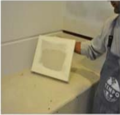
PUTTY SHOULD APPLIED TO THE INNER COVERS BY DEMOUNTING THE COVER
