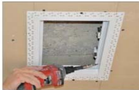
INTERNAL SCREWING VIEW
