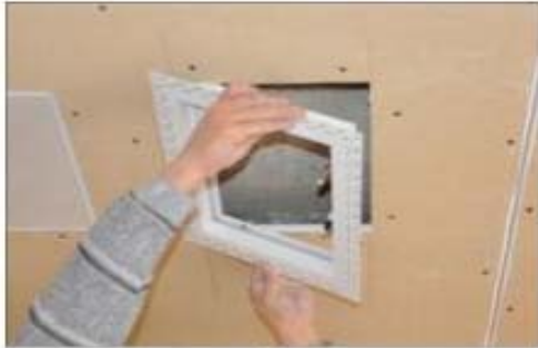
ASSEMBLY OF OUTER FRAME
