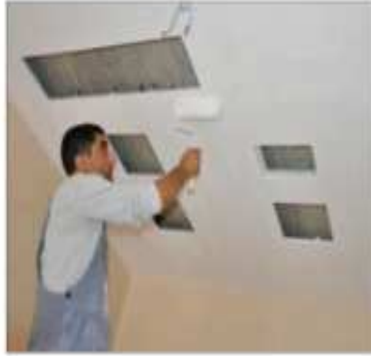
PAINT SHOULD APPLIED TO THE INNER COVERS BY DEMOUNTING THE COVER
