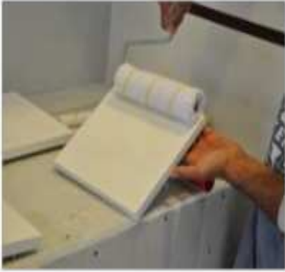
PAINT SHOULD APPLIED TO THE INNER COVERS BY DEMOUNTING THE COVER
