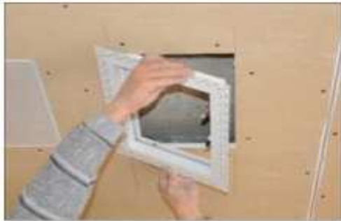
ASSEMBLY OF OUTER FRAME
